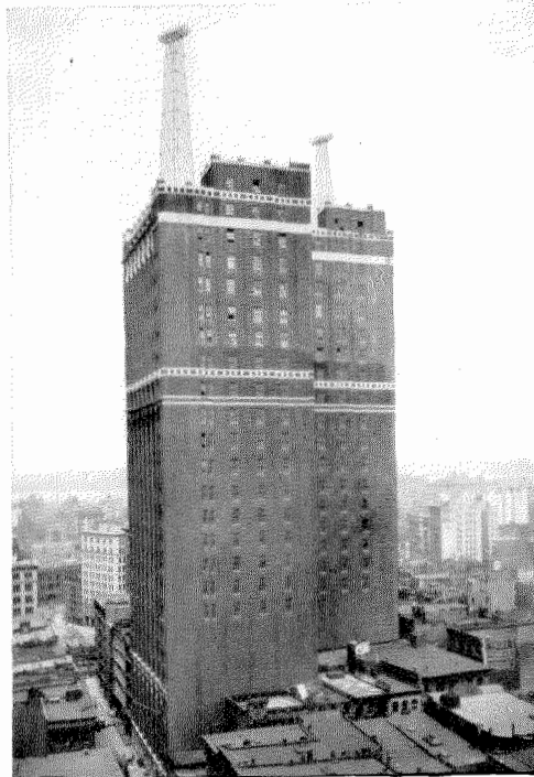
Figure 17—Long distance telephone building, New York City
