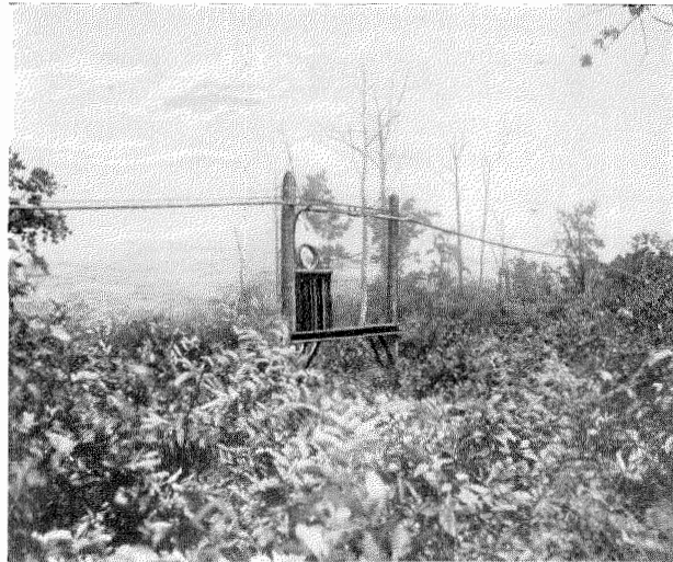
Fig. 8—Toll cable line showing loading coil case
