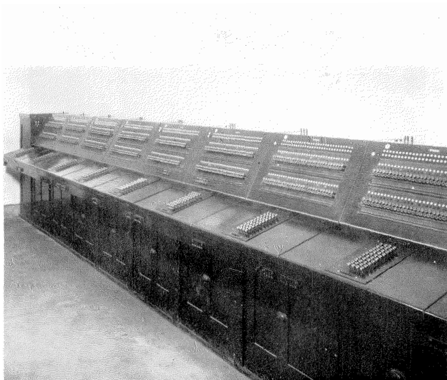
Figure 6—Cordless “B” Positions in Machine Switching Office
